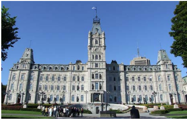
Ill. 1: The Parliament Building in the city of Quebec, Canada.
